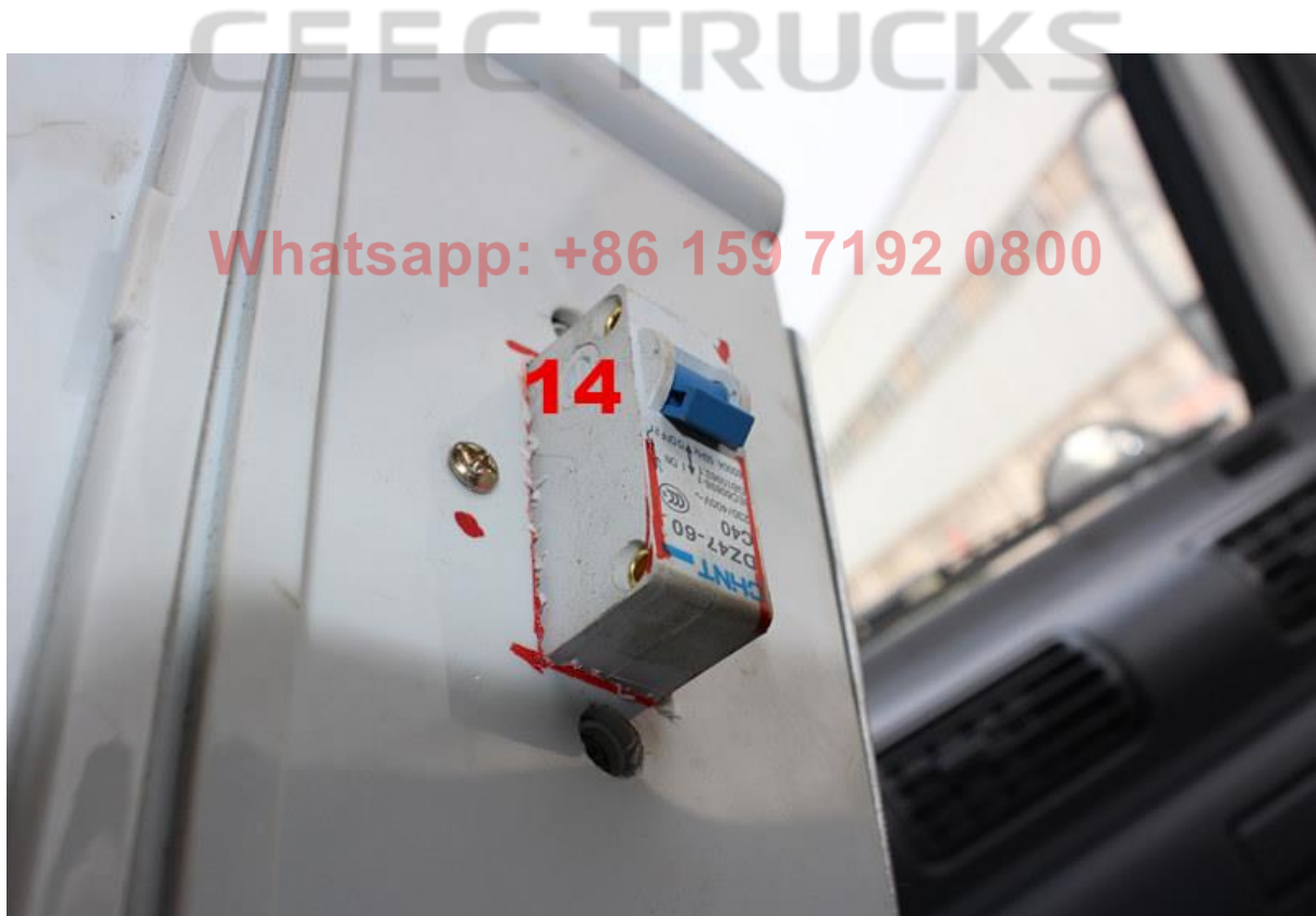
13. Button #14 control Whole Electricity
